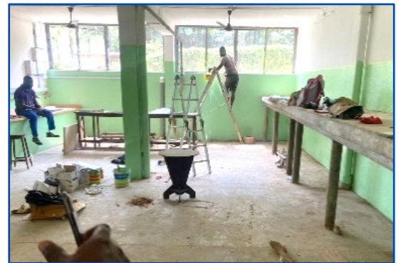
Renovation of new workshop space at the Catholic Conference Centre
