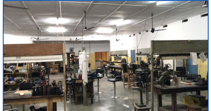
New Workshop Ceiling
